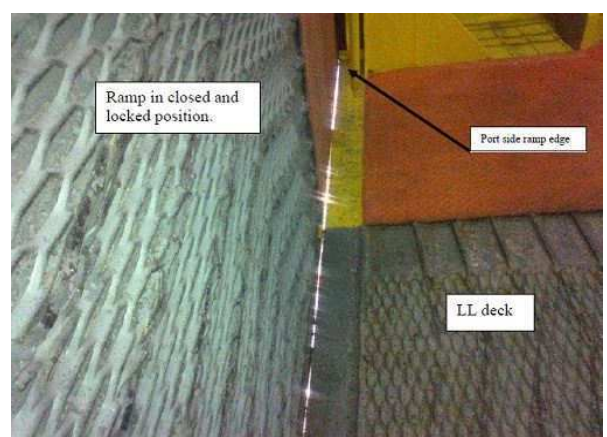
Stern door in closed position: no weather tight due to possible deformation.
