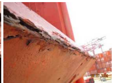
Top portion of door structure wasted and holed
